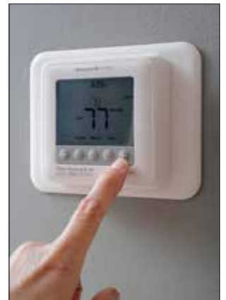
MARK GILLILAND, PIONEER UTILITY RESOURCES
